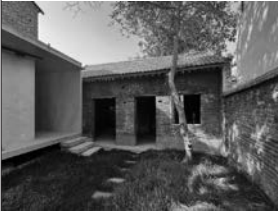
The courtyard and connecting buildings before the renovation.
